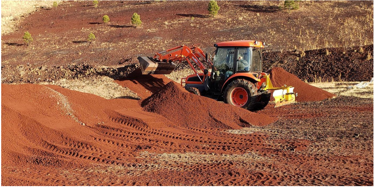
Material then being spread evenly over the face of the berms.
