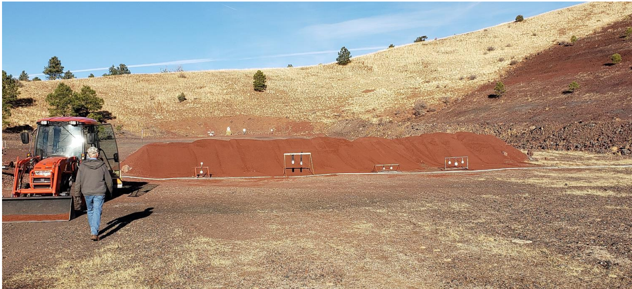
The 100 yard Rifle berm work completed. Thank you Keith!
