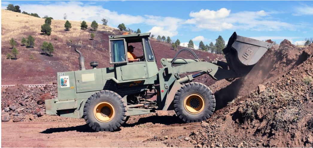
Realigning berms
